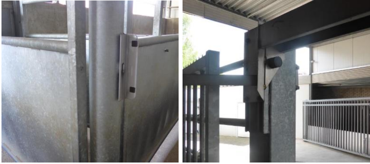
Rubber-stickers and knobs to prevent metal banging to metal
